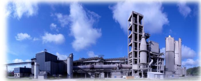
Gargenville plant, France
